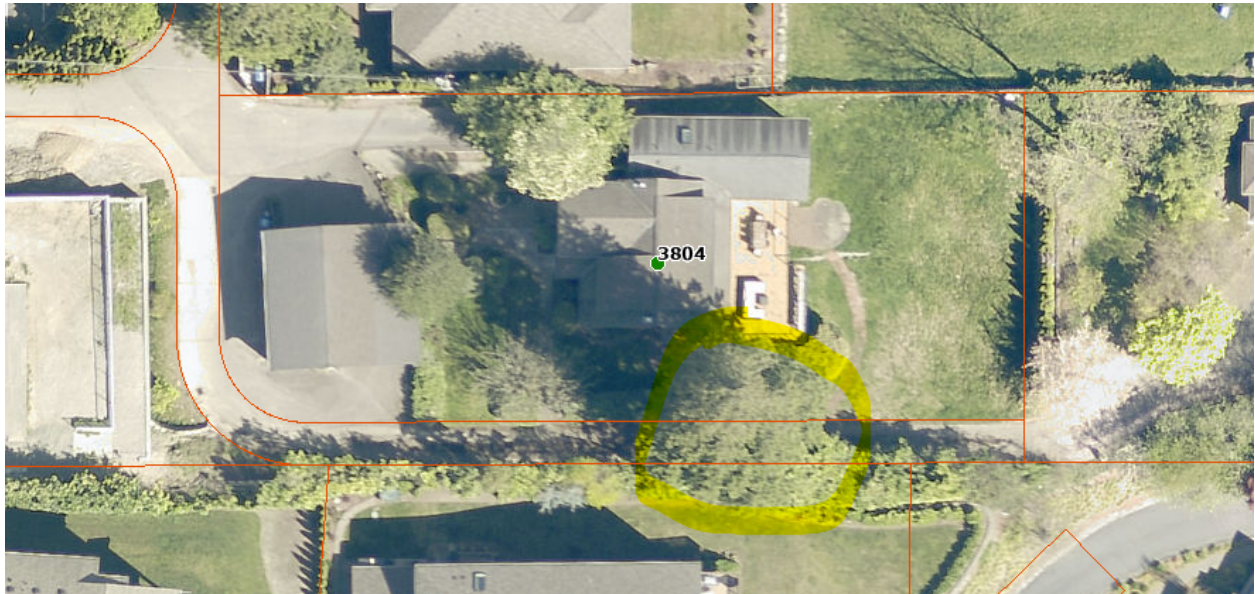
Image 2. An overview of the subject parcel with the previously removed tree circled in yellow.
